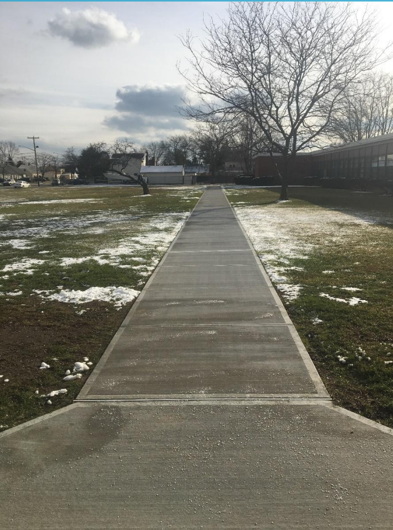
Concrete Path at Gardiners Avenue
